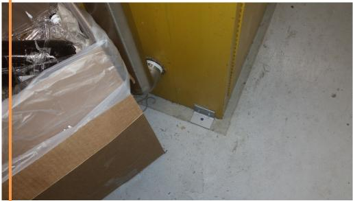
Se ismic restraint on supply cabinet
