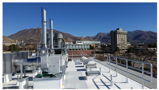
Guard rails and stack bracing on roof
