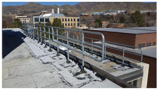
Guard rails installed on roof
